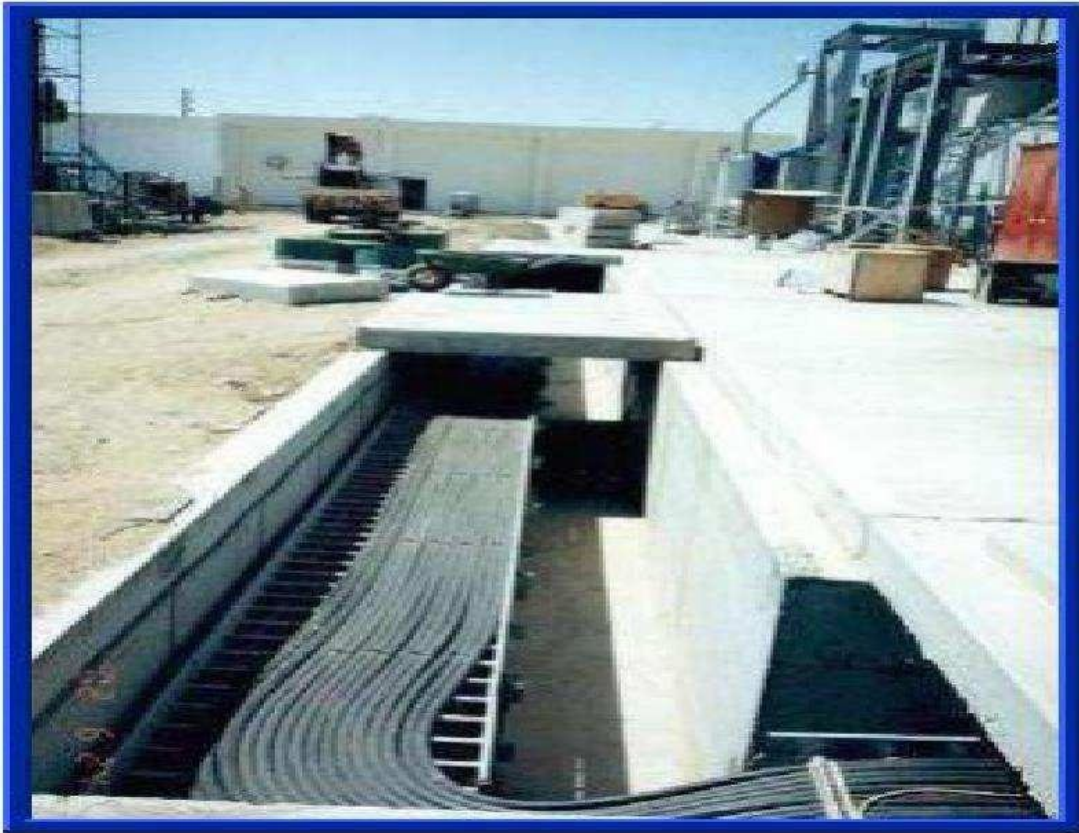
SUBCABLE ELECTRICAL SYSTEMS WORKS
